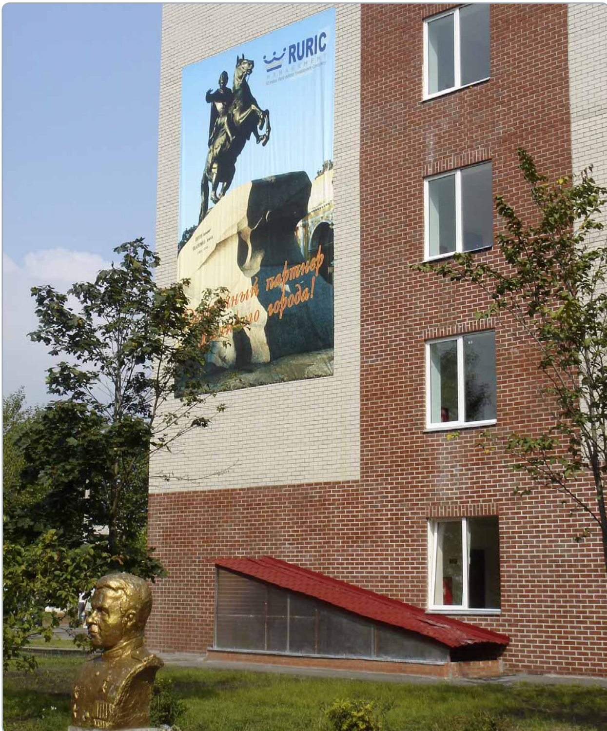
Replacement building for the Russian army in Petrodvorets: barrack for cadets.
